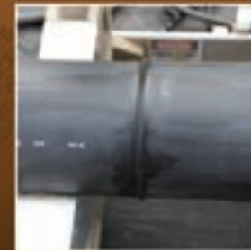
Welded areas of pipe are stronger than the pipe itself
