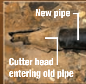
Old pipe is burst and new pipe is installed at the same time
